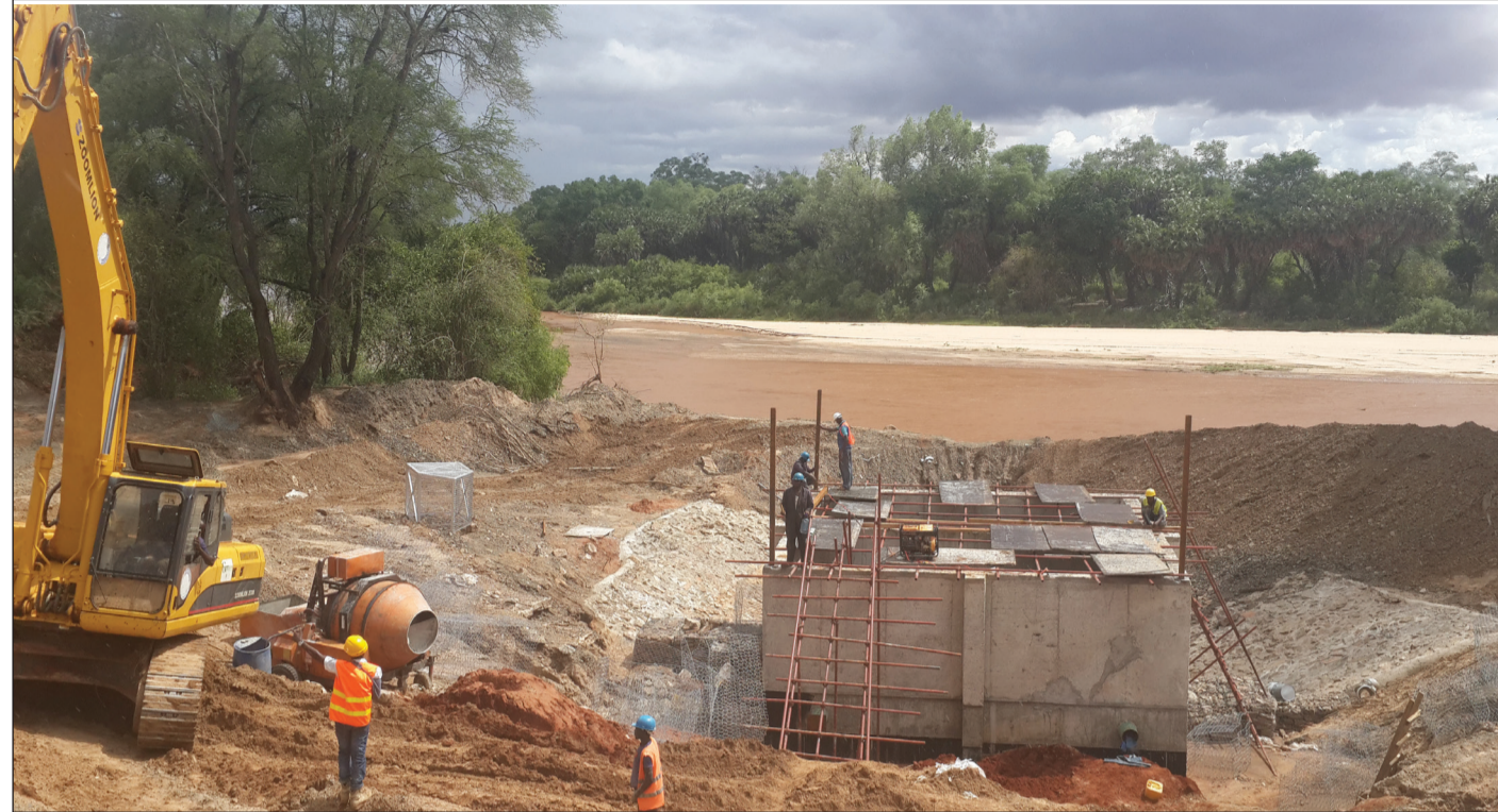
A section of workers at the point where water from River Galana will be pumped through to the farms. PHOTO: EAGC-RATIN
