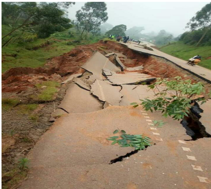
Plate1: Road connecting Rwanda and Uganda through Gatuna Border (20/5/2018).
